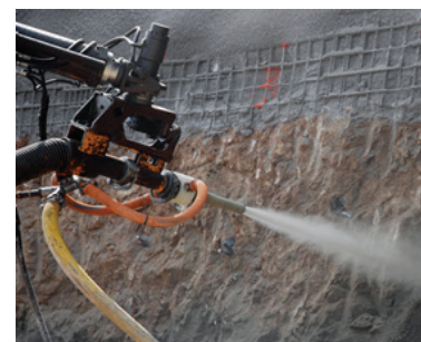
TESTING THE WORKABILITY AND THE SPRAYABILITY OF THE MATERIAL
