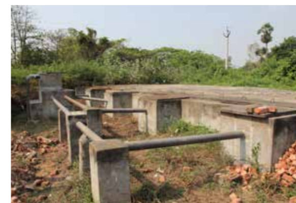
Construction of the HPAS system
