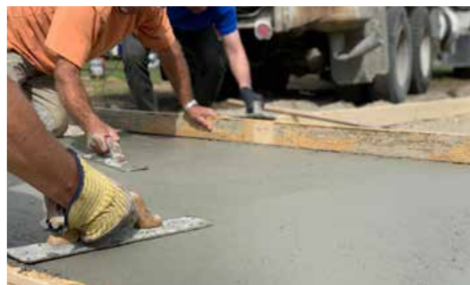
Laying the pavement
