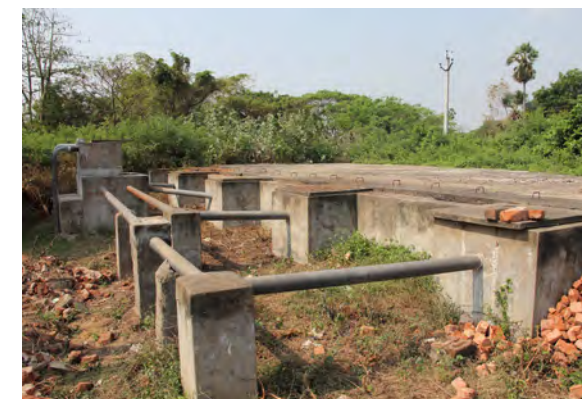
Construction of the HPAS system
