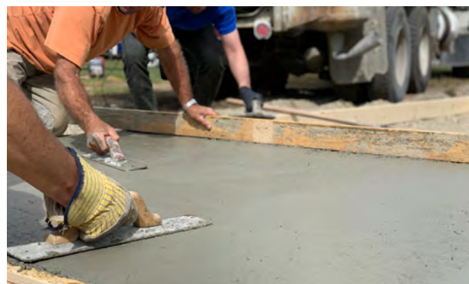
Laying the pavement
