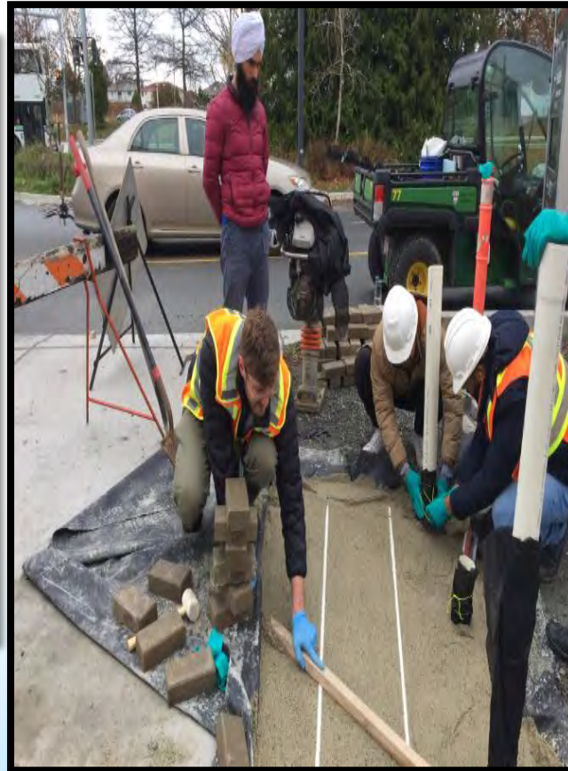
Bedding Soil Placement
