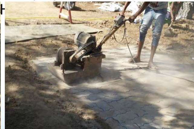
(l) Compaction on paver blocks
