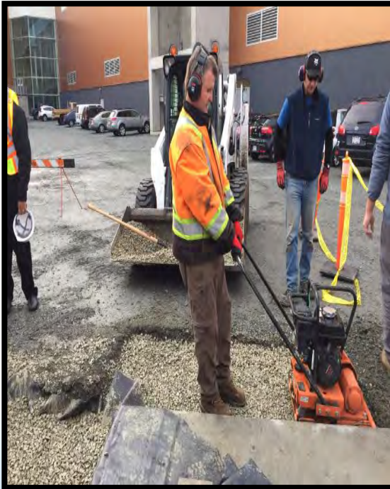
Gravel Compaction
