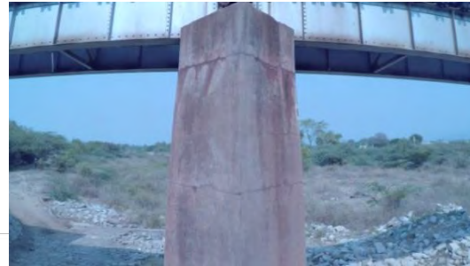
Renigunta Railway Bridge, India
