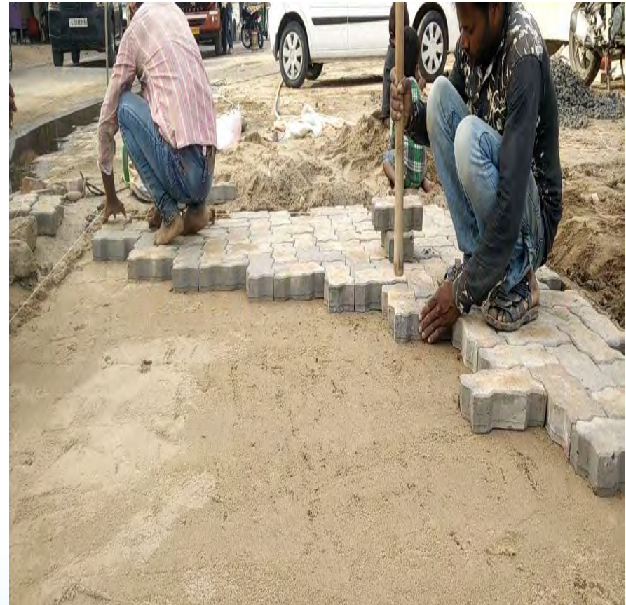
Laying of Paver blocks having depth of 60 mm in Herringbone Pattern
