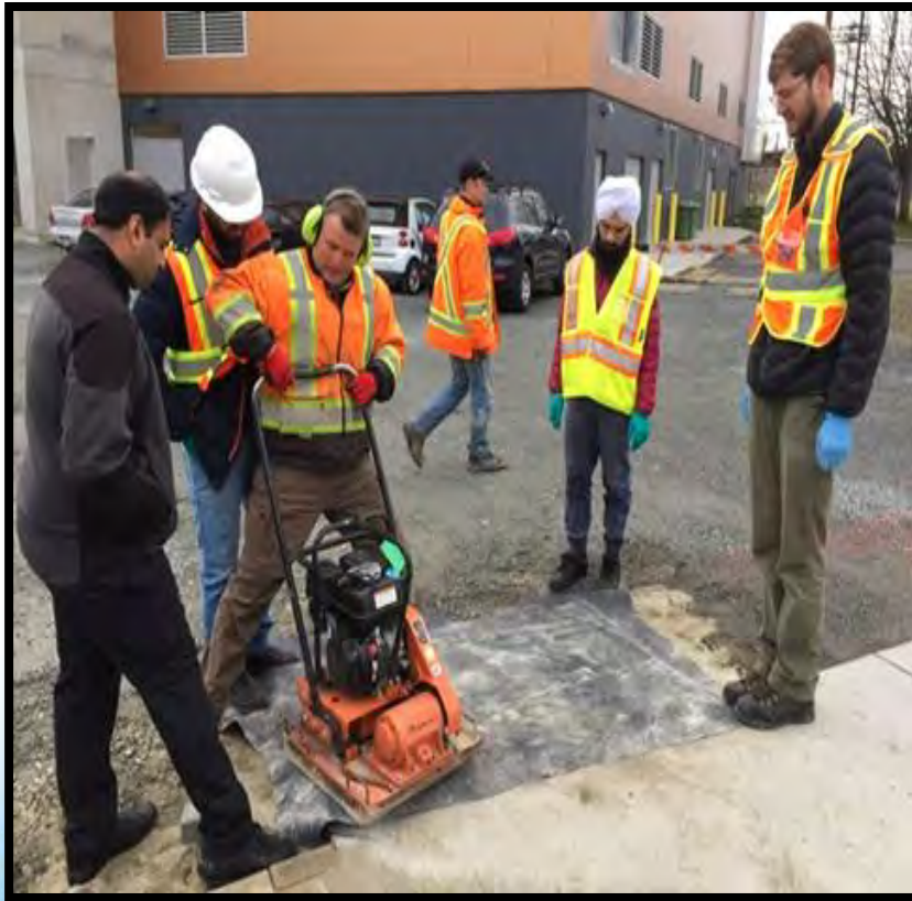
Final Compaction
