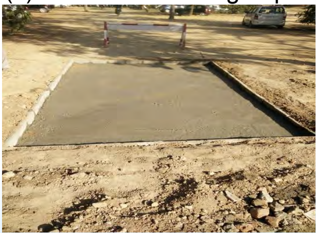
(f) laying of PCC having depth
