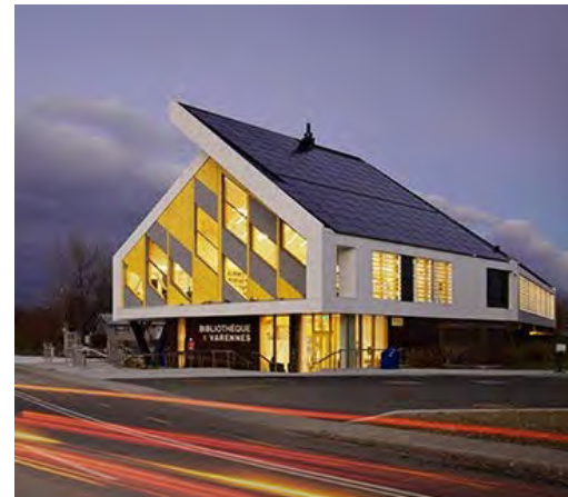
BIPV/T roof on Varennes Library
