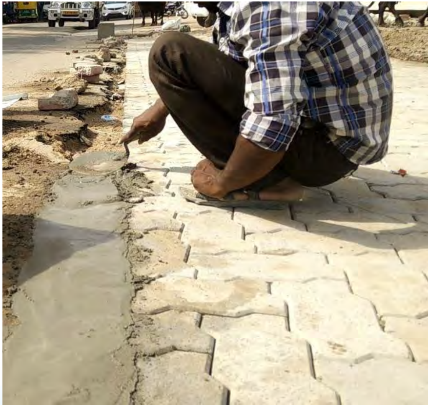
Mortar filling between boundary of paver blocks & kerbing
