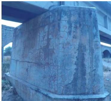
Ponnier Railway Bridge, India
