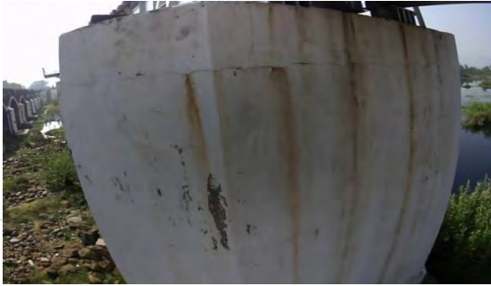
Nagari Railway Bridge, India
