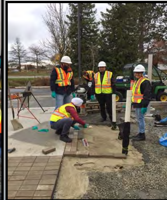
Paver block placement
