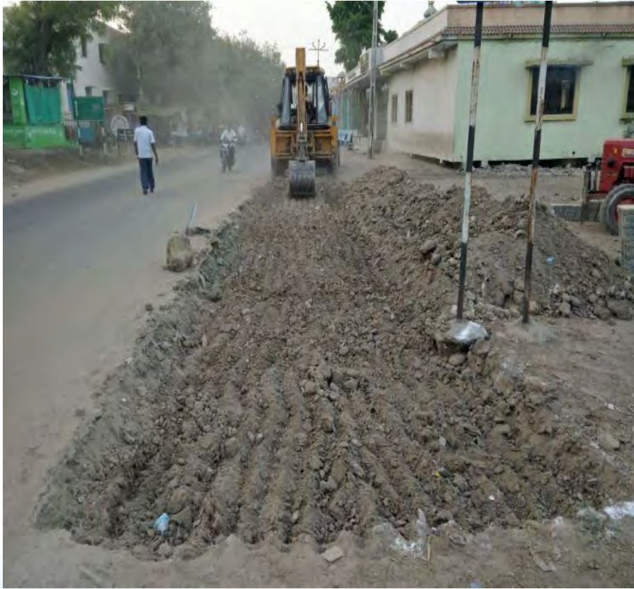
Excavation of size 2.5 m × 16 m having depth of 200 mm using Backhoe
