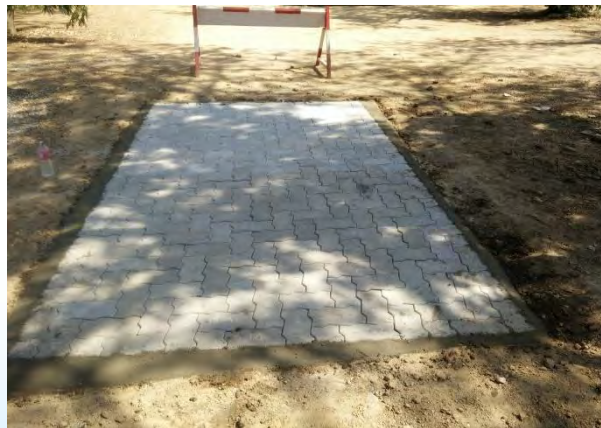
(k) Paver block Pavement Stretch
