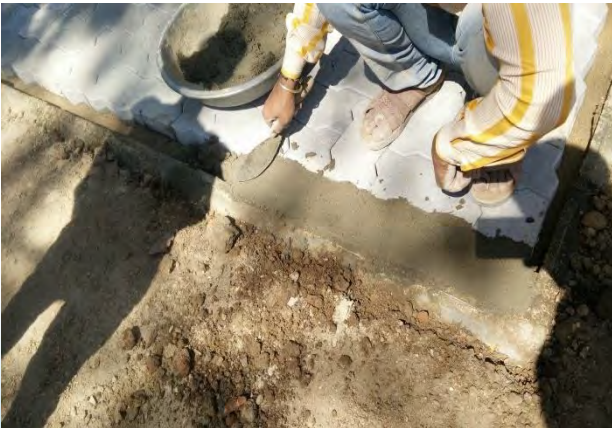
(j) Mortar filling near edges
