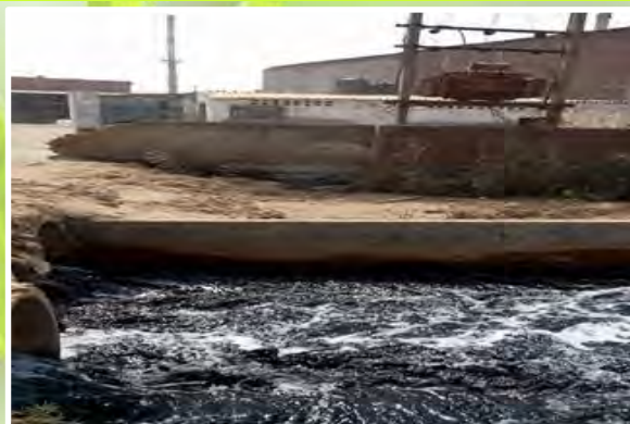
Industries disposing effluent into drain.
