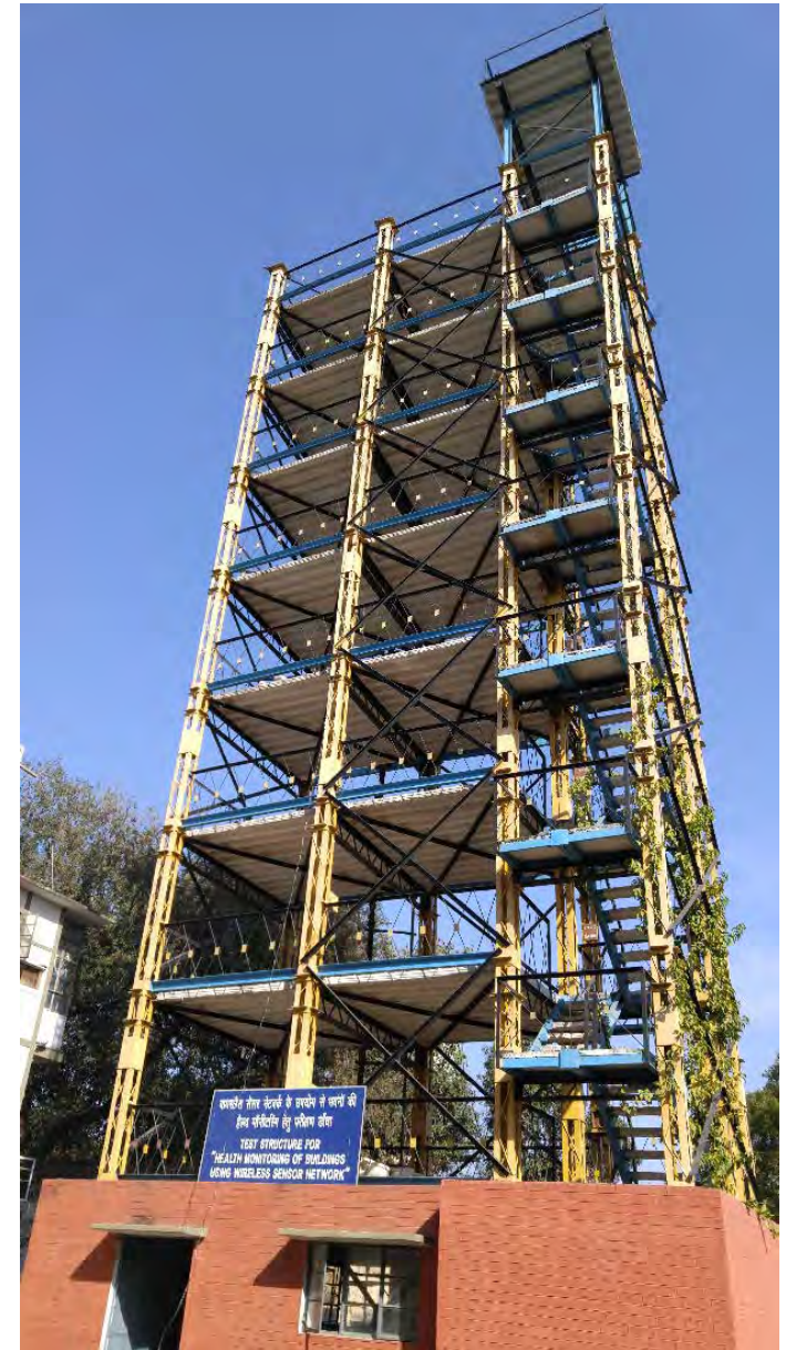
Eight Story Steel Building in CSIR-CBRI Roorkee
