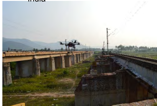
Ambur Railway Bridge, India
