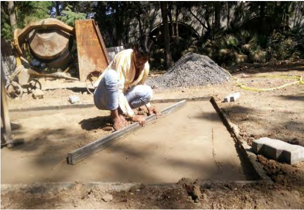
(g) Laying of 40 mm sand
