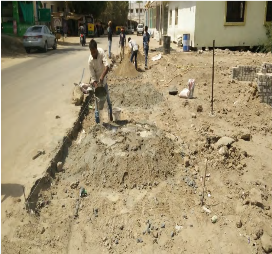
Preparing of Plain Cement Concrete
