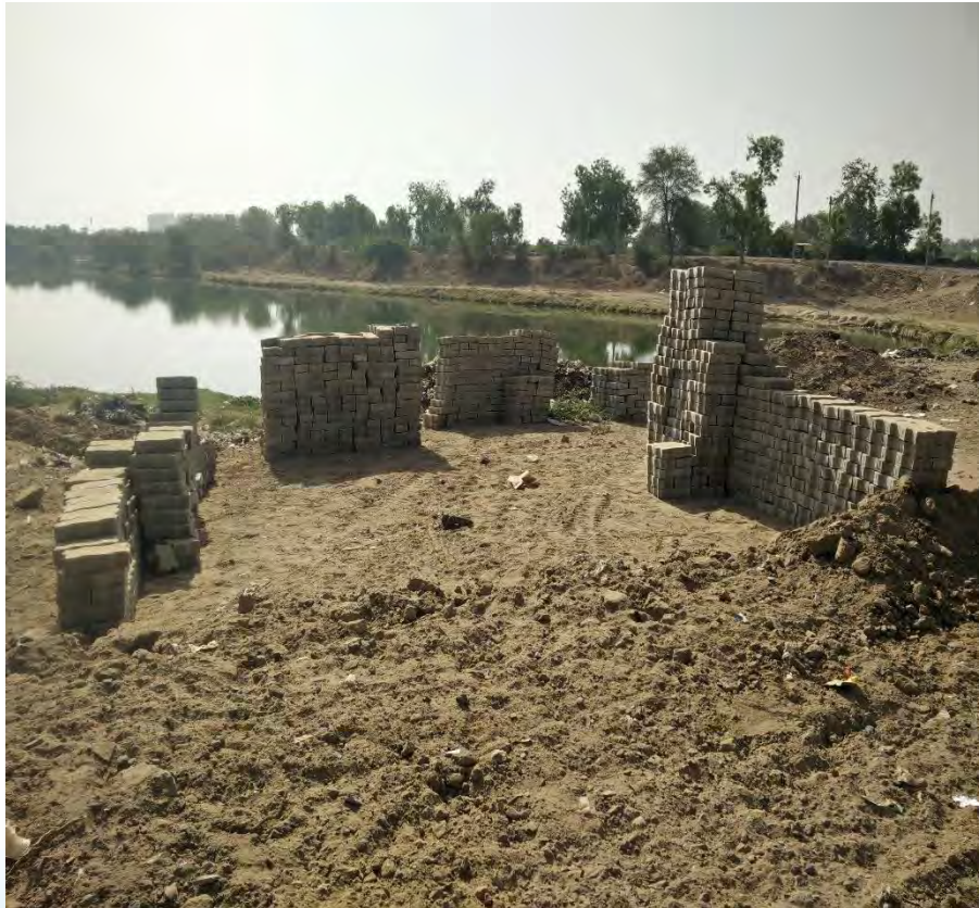
Storage of Alkali Activated Concrete Paver Blocks at Pavement Site
