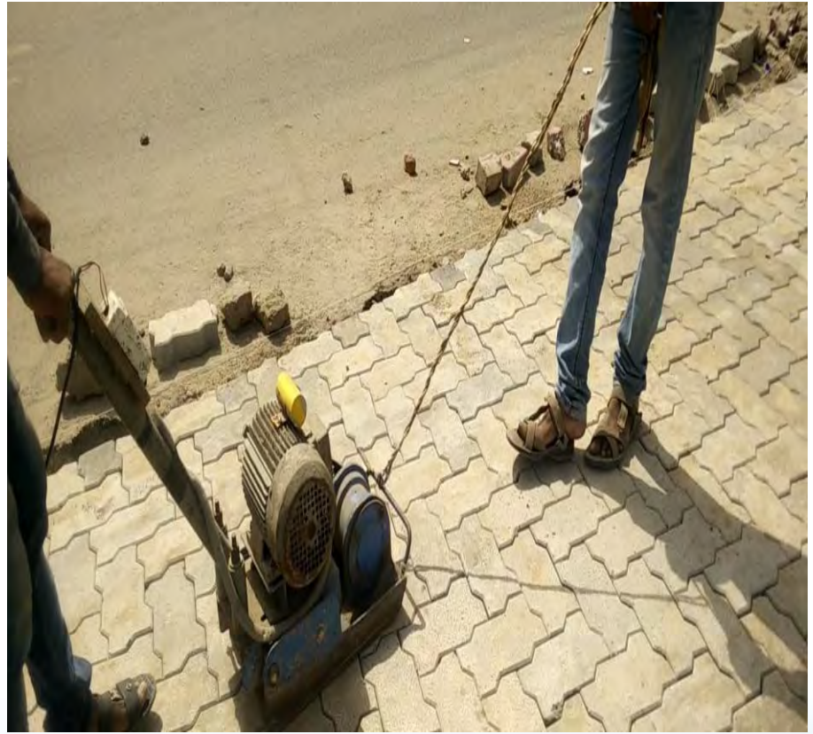
Joint sealing between paver blocks using compactor
