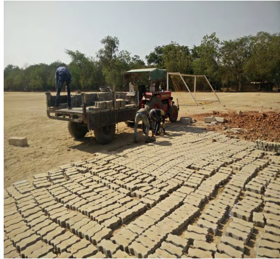
Transportation of Alkali Activated Concrete Paver Blocks to Jaspur Village Site
