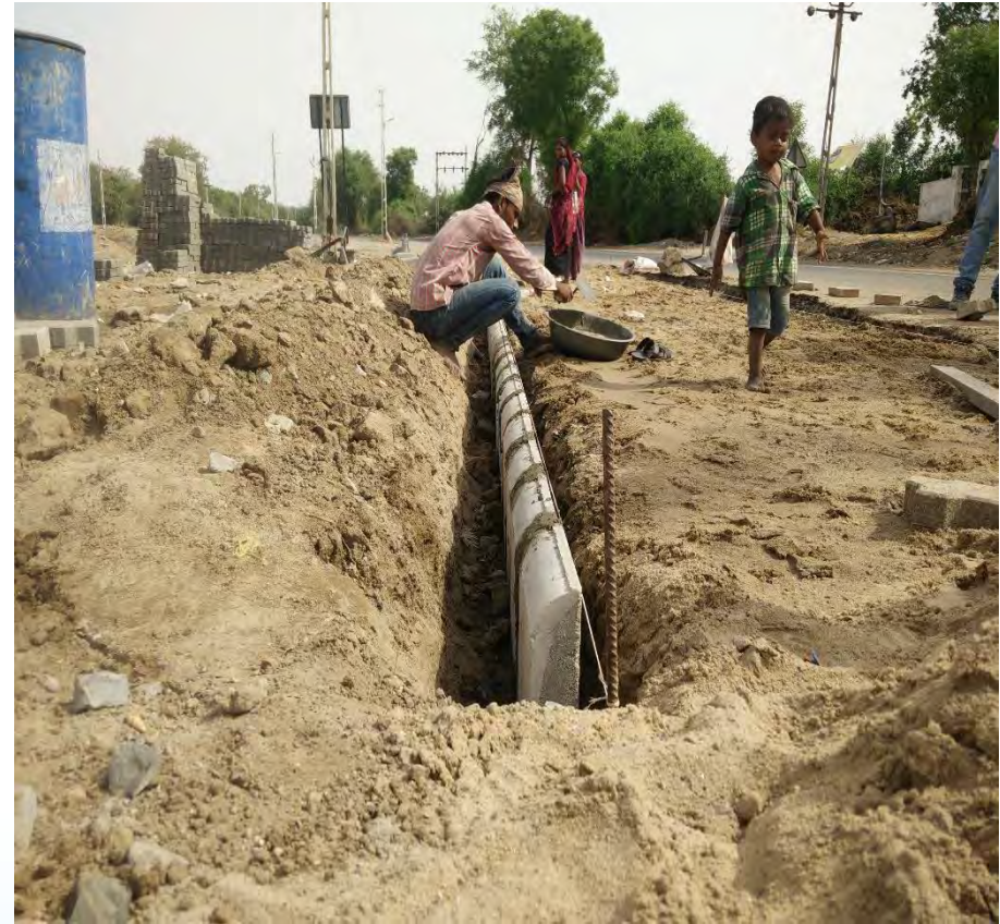
Laying of 12 inch kerbing around edges of rural pavement
