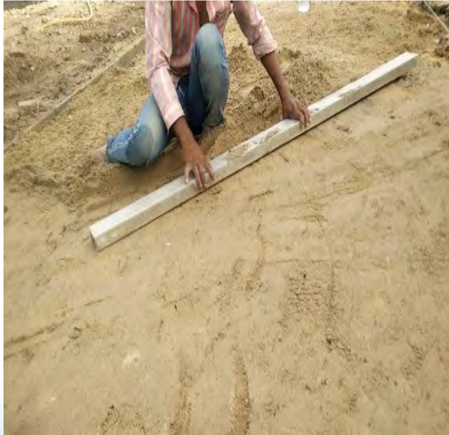
Laying of 40 mm depth sand bedding & levelling
