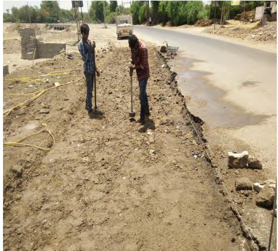
Compaction & Levelling of Earth in Progress at Pavement Site
