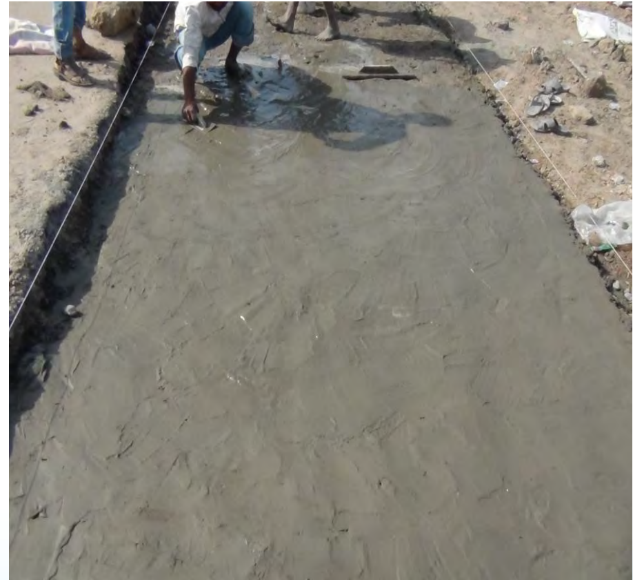
Laying of PCC of depth 100 mm
