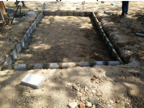
(e) laying of 9 inch depth Ker
