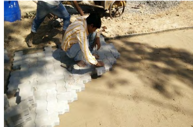
(i) Laying of Pavers in
