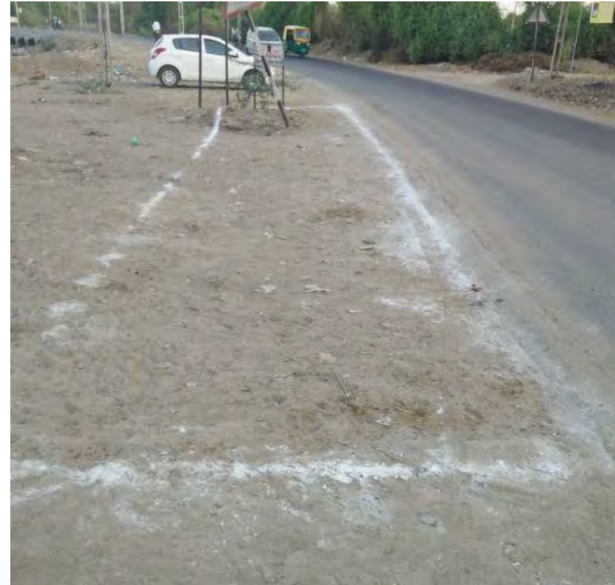
Marking of Required Excavation having Size of 2.5 m × 16 m on Proposed Pavement
