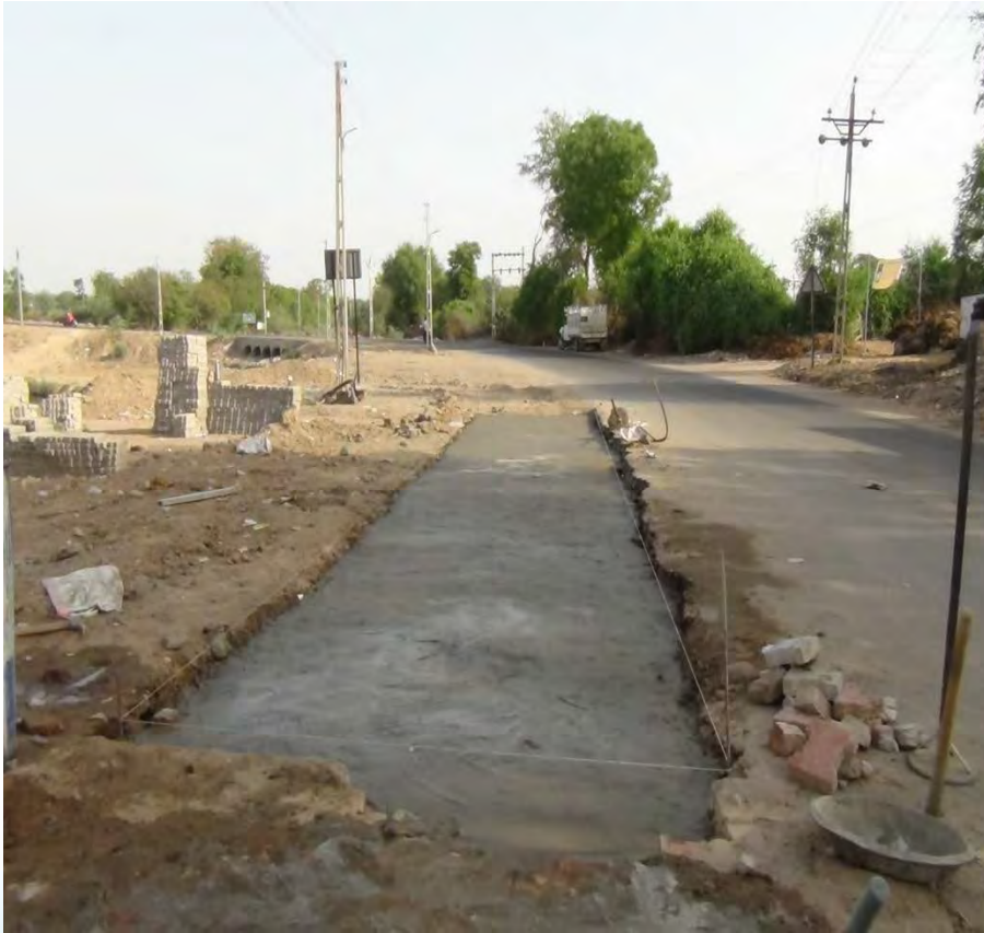
View of Pavement after completion of the PCC work
