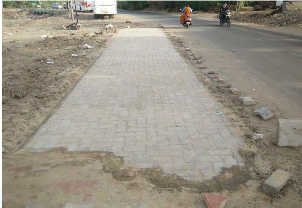
Actual image of Rural Pavement at Jaspur Site
