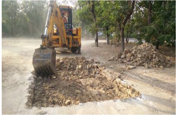
(c) Excavation having depth of
